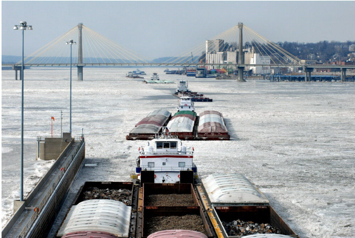
Figure 12: Tows delayed during ice conditions, Melvin Price Locks and Dam, Mississippi River, February 2007; ice build-up in the lock caused one tow to become stuck, temporarily shutting down the lock; later, width restrictions were implemented (from PIANC, 2008; photograph by Russell Elliott, US Army Corps of Engineers)
